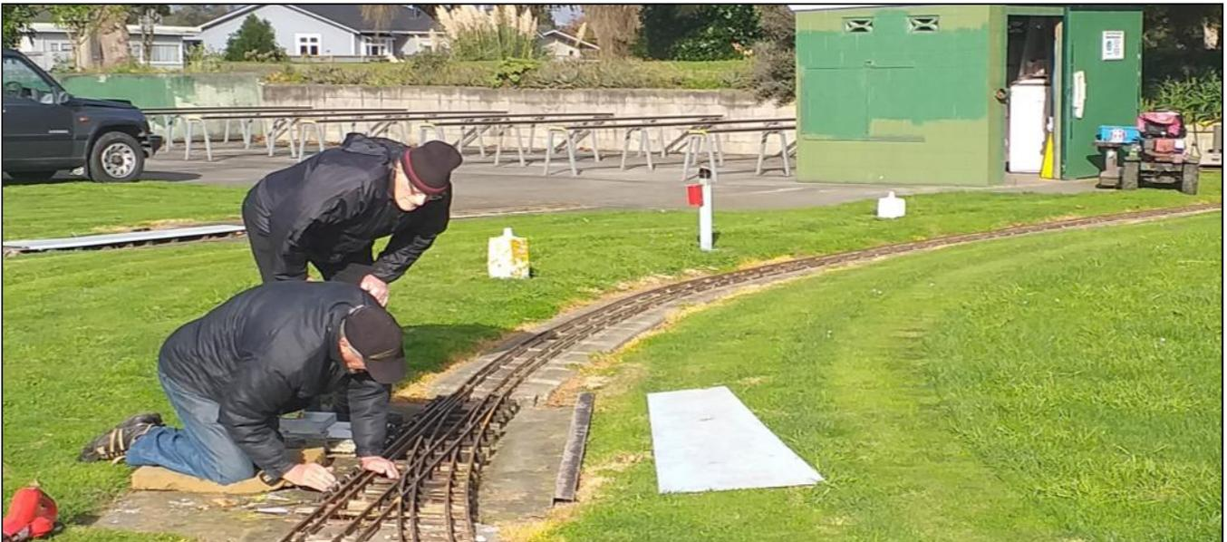
Ian McLellan and Doug Chambers servicing one of the railways holder style turn-outs, cleaning, lubricating and adjusting the blade alignment if necessary paying particular attention to the blade alignment. I suspect with Doug's new southern railway "Schools Class " soon to try out a full lap of the Marriner Reserve railway they were paying particular attention to the 3.5 inch gauge.
